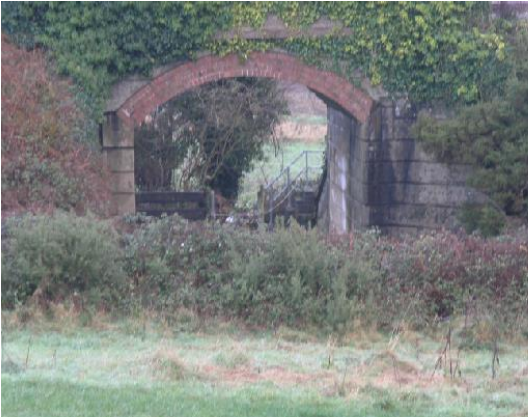
Figure 10.19 Proposed crossing under railway via sub-railway-line bridge
