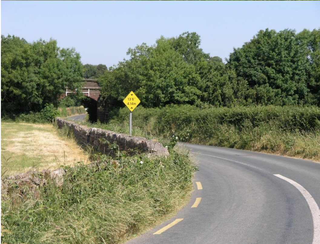
Figure 10.22: Dunbrody Bridge and Railway Bridge
