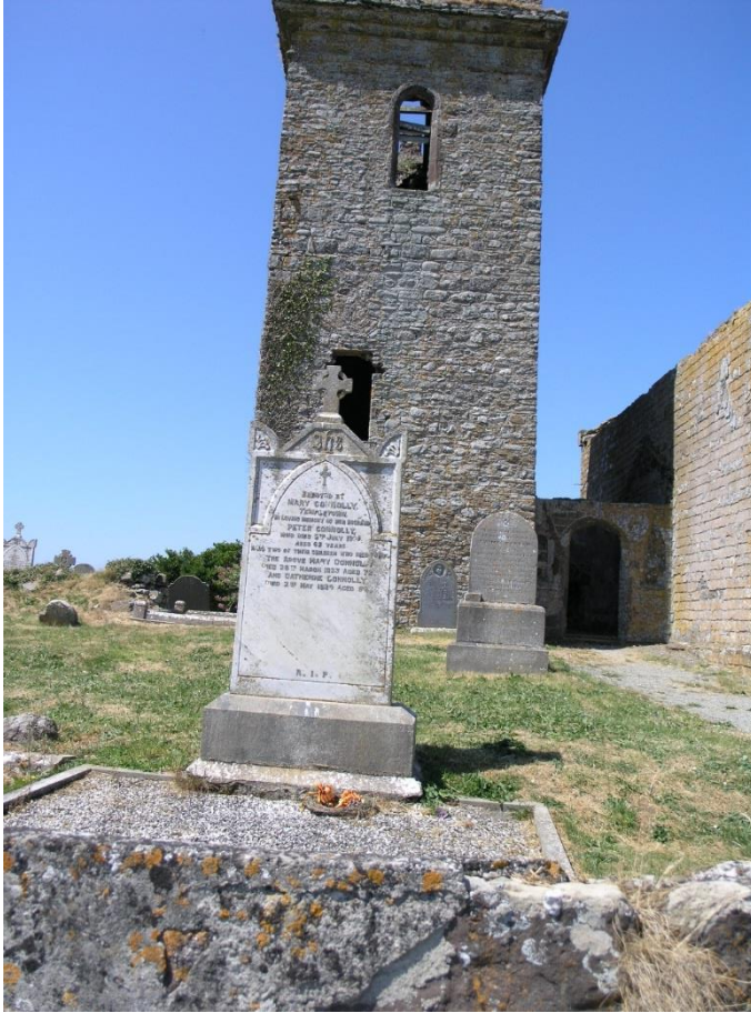
Figure 10.5: Fourteenth-century Tower (RMP-WX-049-008) at Templetown
